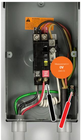
If measurements 1 - 4 are inaccurate, the service voltage is faulty. Call an electrician. If the measurements are accurate, go to step 4.
