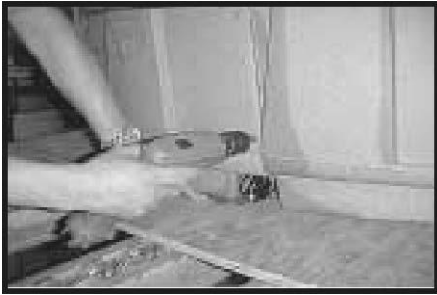
Remove & save access panel screws. Use caution when reinstalling the screws. Do not overtighten.
