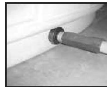
Suggested sample of installed junction box. Route incoming power through the shell's
