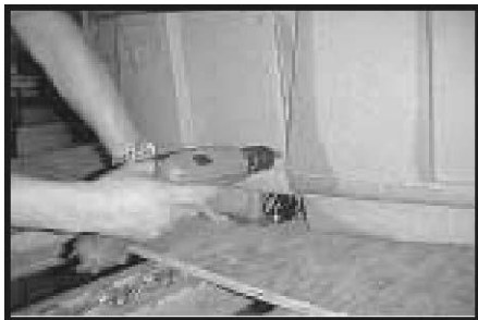
Remove & save access panel screws. Use caution when reinstalling the screws. Do not
